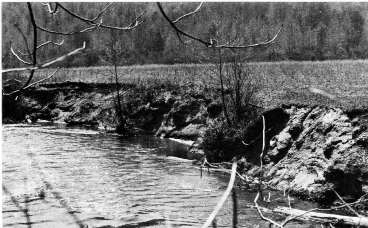
Eroding river banks along the West Fork.
