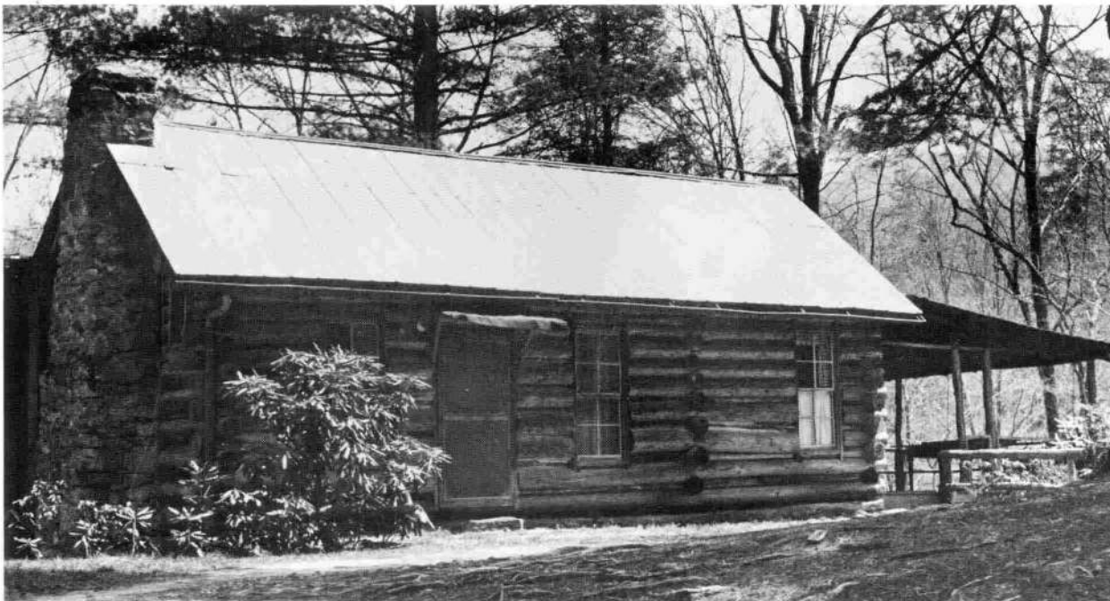
A summer home in Section I. Rustic design is compatible with scenic classification.
