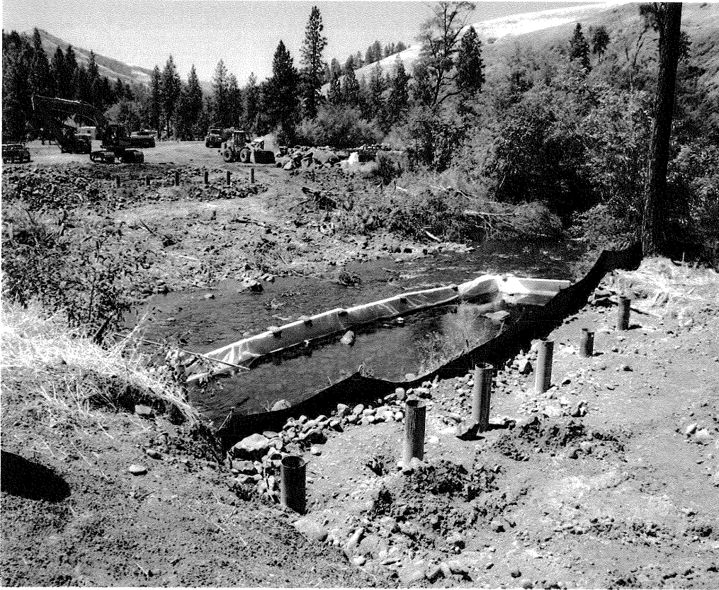
Figure 4. Photo of a similar work area isolation structure on the Umatilla River.
