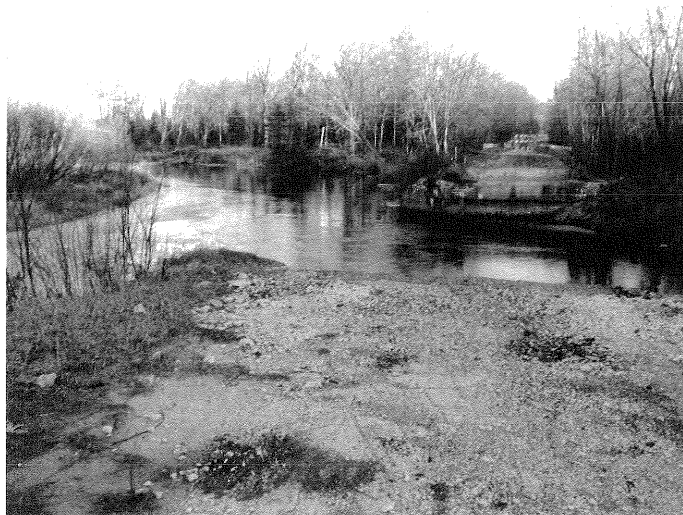
Figure 3: Constriction of the Sturgeon River by bridge abutments installed circa 1917. Bank scour upstream of bridge can be seen at left middle ground and on the opposite side of the river, upstream of bridge abutment. Flow is from left to right.
