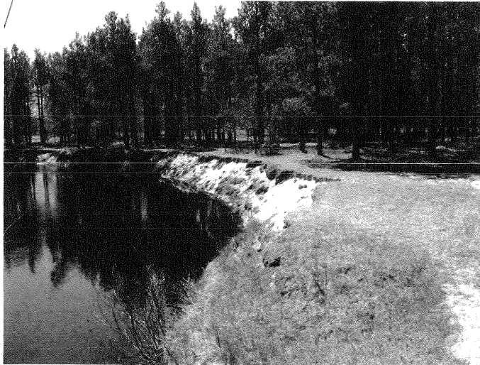
Figure 4: First Meander Bend immediately downstream of the proposed project site. Inadequate span of original structure likely contributed to bank erosion of the deep, droughty, infertile sands adjacent to the river.
