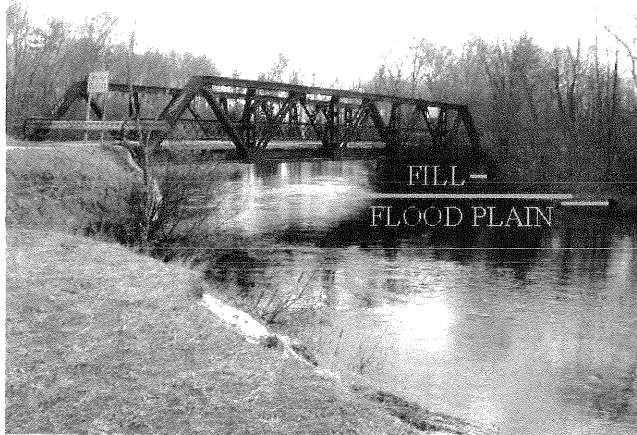
Figure 9. Existing approach on the eastern side of the Sturgeon River is fill material that extends into the flood plain. This approach will still constrict the Sturgeon River after project completion. However, the new structure would have a greater hydraulic capacity and provide for a much improved, though not completely unaffected, flow regime through the area.
