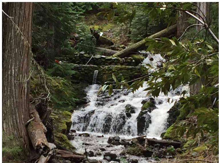
[Left to right] 1. Lake Creek water intake. 2. The water intake creates a diversion on Lake Creek that spans only part way across the creek. NPS photos.
