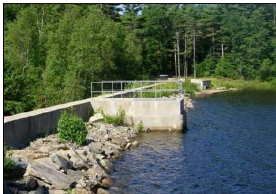
Middle Pond Dam. Photo: Unknown
