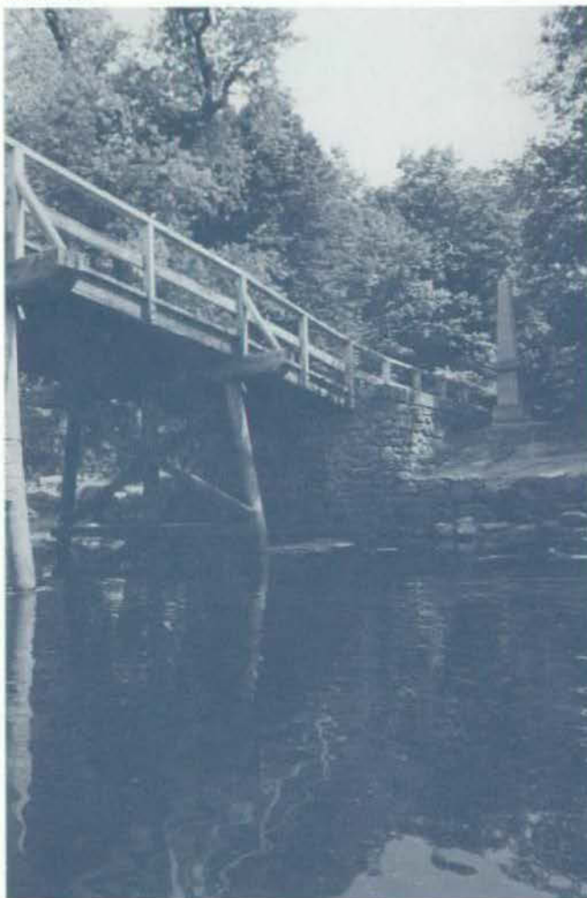
North Bridge, Concord.
