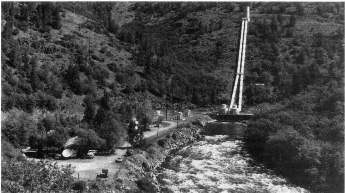
J.C. Boyle Powerhouse.
