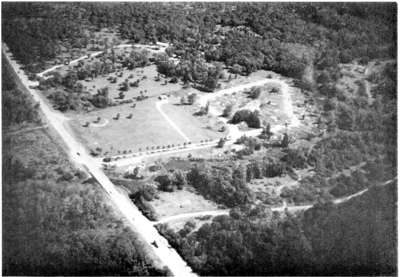
River Mile 13.5 - Palm Beach County has Purchased a 187-Acre Site Along the Loxahatchee River at Indiantown Road. The County Removed an Existing Trailer Park and Plans to Develop the Site as a Passive Recreation Park Focused on the River
