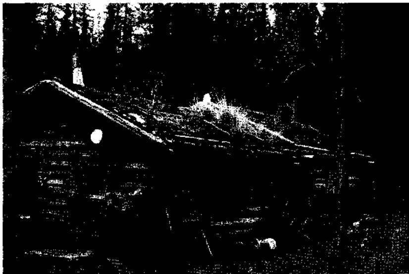
Photo 3. Local area residents sometimes build cabins in association with hunting, trapping or other subsistence activities. Designation would formally recognize the cultural value of these structures.
