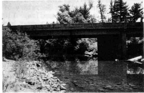
Highway 199 Bridge Across the West Fork.
