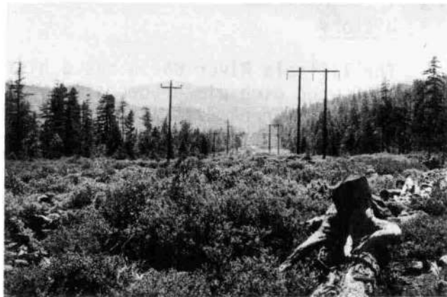
Transmission Line Near the West Fork.
