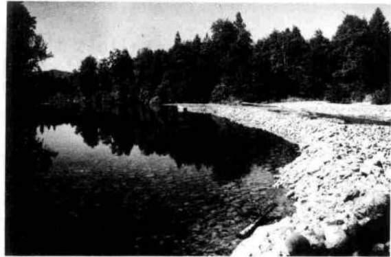
Gravel Berm Used to Divert Irrigation Water.
