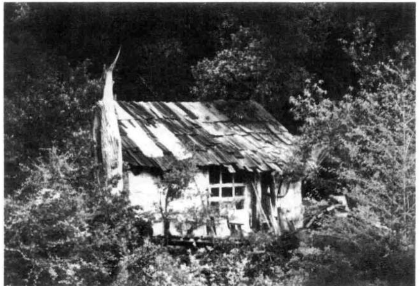
Cabin at Clear Creek Adds Historic Touch.
